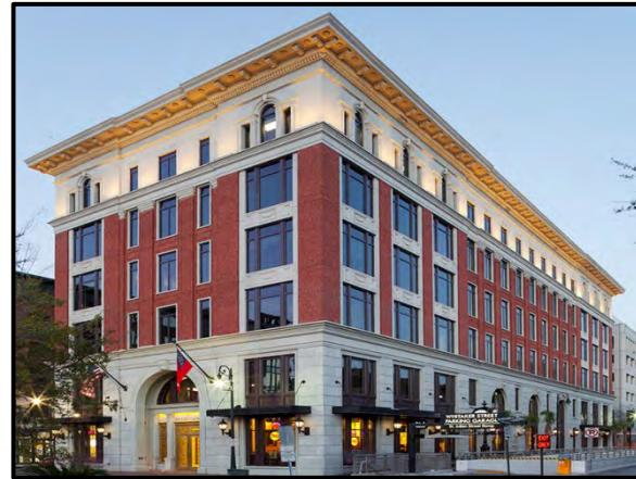
*A significant amount of glass is provided at the base of this building. The base also reflects a greater height than any single floor in the middle. Note the step back on the top floor.*
