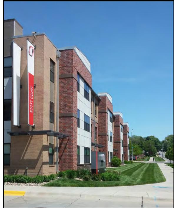
*As above, this building utilizes articulated walls, columns, changes in roof height. Yet it also utilizes shade structures, balconies and awnings to help break up the mass.*
