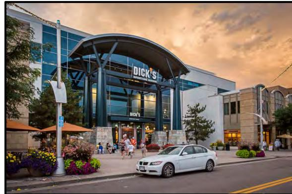
*This single-story large format retail building appears to be multi-story, is located adjacent to the street, and has facades that contain display windows and pedestrian-scale construction material.*
