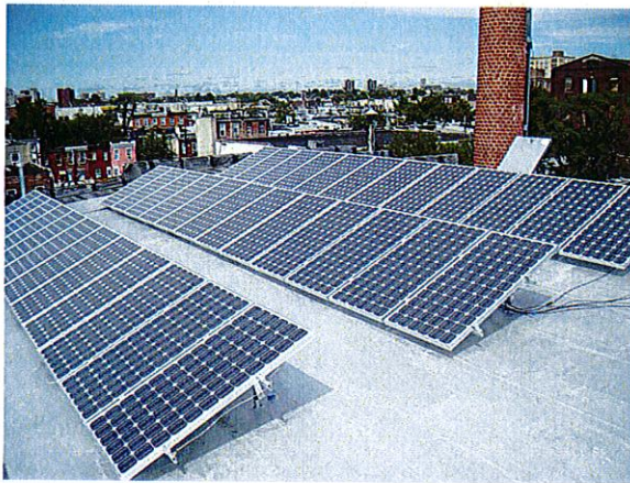
Roof top application of an older building in Philadelphia.
