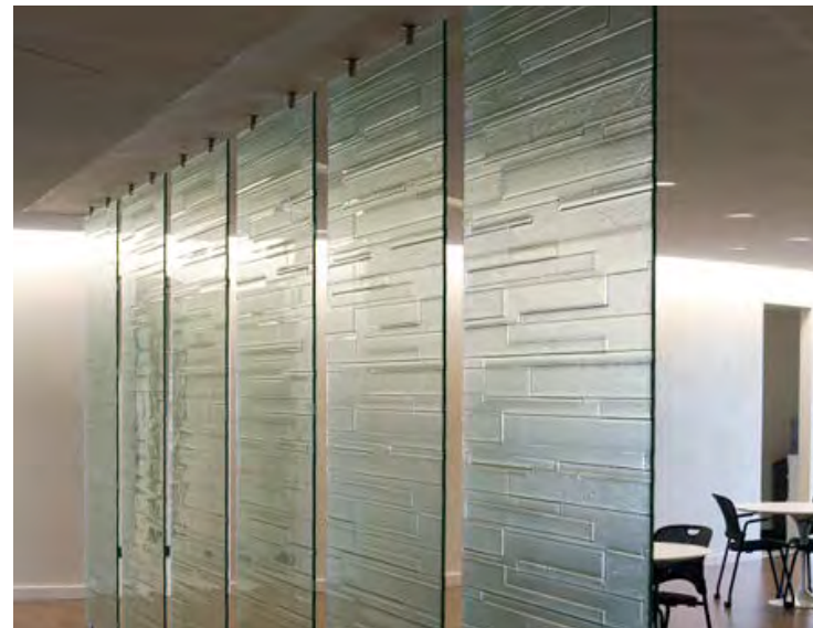
Textured etching on front side of glass, frosted vinyl applied to flat back side.
