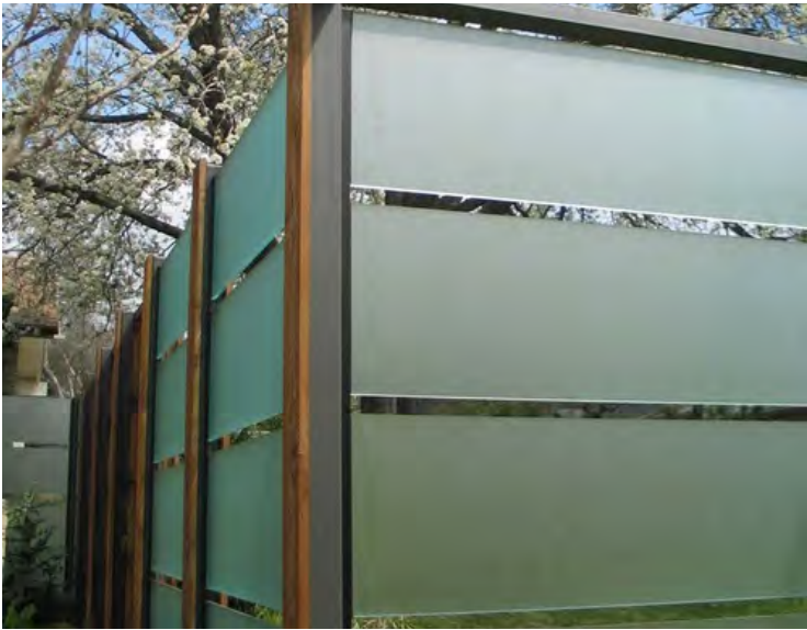
Close up detail of frosted glass panes in a custom metal and wood enclosure in use as a fence around a residence
